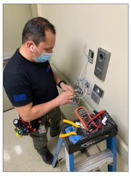
entrance for EMS crews, and remote door releases were provided for use by security staff. The overall project included CSI providing all new *Salto Systems* access control which was integrated with *Aiphone* IP intercoms, this included all new cabling and other related hardware.
